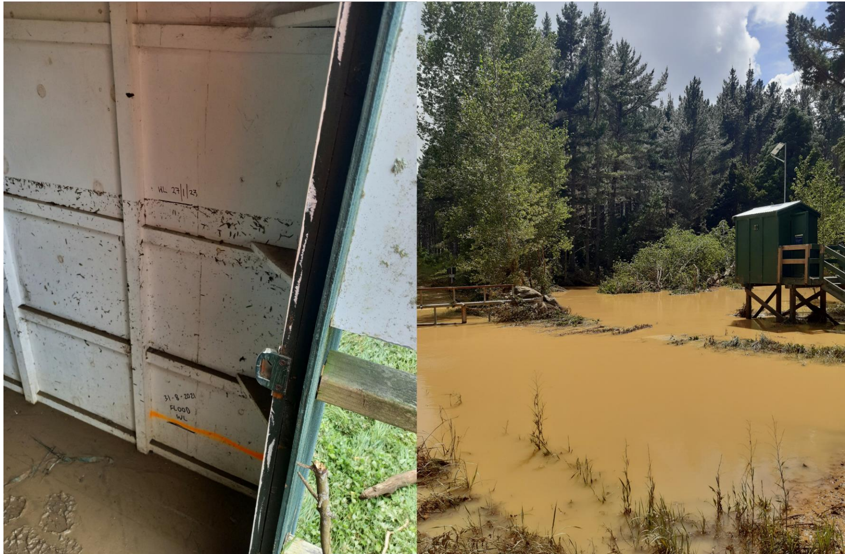
Figure 18. Left image shows flood marks inside instrument shed at Kaukapakapa following Auckland Anniversary event in January 2023. Right image shows the instrument shed at Kōurawhero which was also flooded in the Auckland Anniversary event. Source: Photos provided by Auckland Council (EEMU) Hydrology team.
