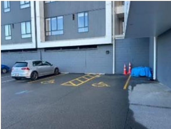
Figure 82: Unallocated accessible parking at apartment building (P8 AP)
