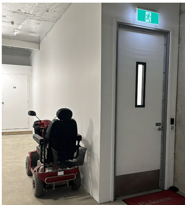
Figure 26: Mobility scooters stored in underground carpark (P8 AP)
