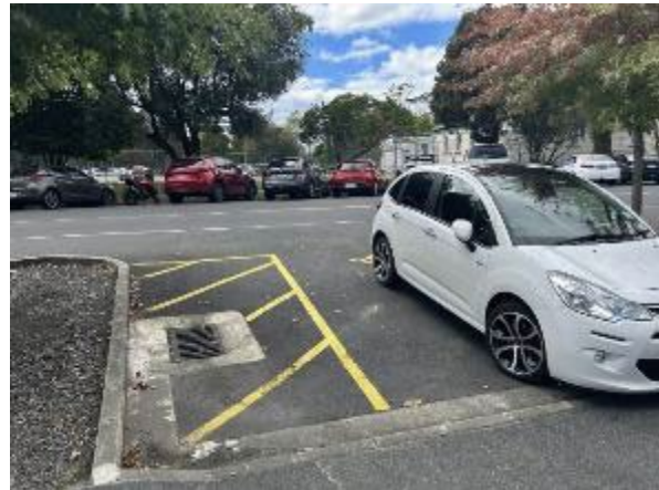
Figure 83: Unallocated accessible parking at apartment building (P1 AP)
