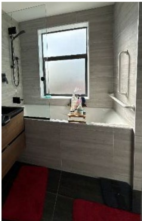
Figure 71: Grab rails added by shower over the bath (P7 TH)
