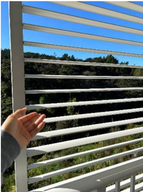
Figure 76: Louvre fins being adjustable (P5 AP)
