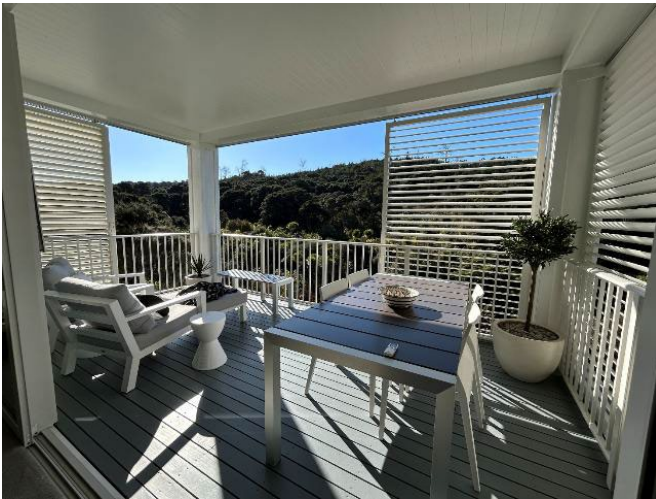
Figure 76: Louvre fins being adjustable (P5 AP)
