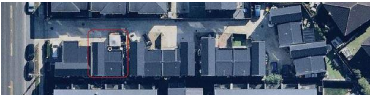
Figure 62: Aerial image of participant's house within the development (P4 TH)
