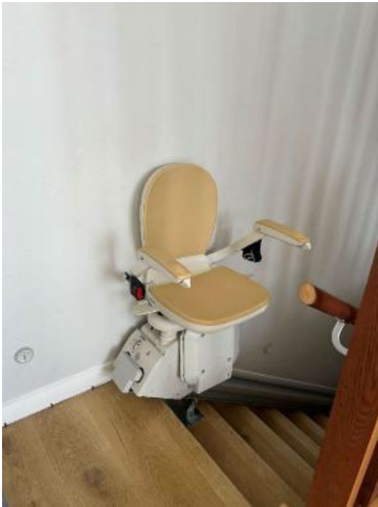
Figure 73: Stairlift (P7 TH)
