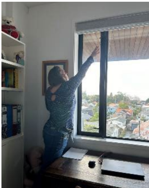
Figure 55: High latch to open window in a bedroom (P8 AP)
