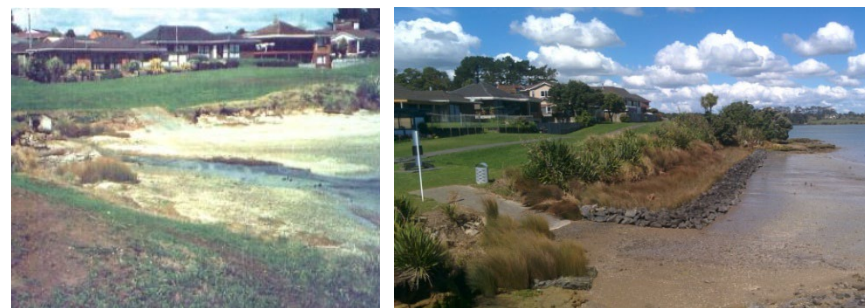
Figure 4-6: Left. St Annes Crescent in 1993 (T+T, 2009). Right. St. Anne's Crescent salt marsh restoration. Note the planted vegetation between the foreshore and the rocky outcrops
