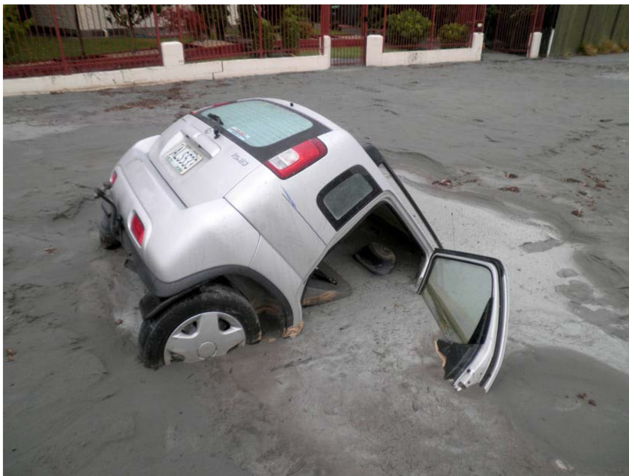
Figure 2: Liquefaction caused by the 2010–11 Canterbury earthquakes created large holes in streets around Christchurch. This car toppled into a hole near Shortland Street in the suburb of Aranui following the 22 February 2011 earthquake. Source: Te Ara (the Encyclopaedia of New Zealand)
