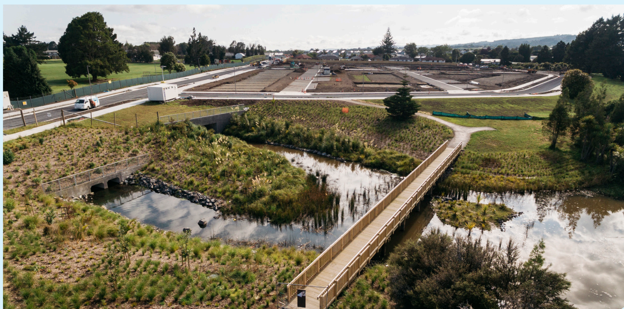
▲ Awakeri Wetlands and Grove Road Box Culvert
