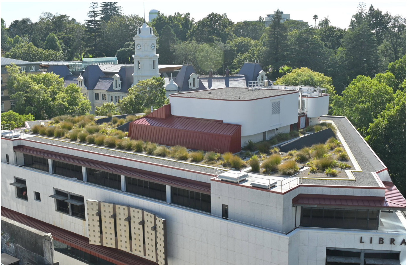
Figure 3: Auckland Central Library living roof Source: Timescapes Limited
