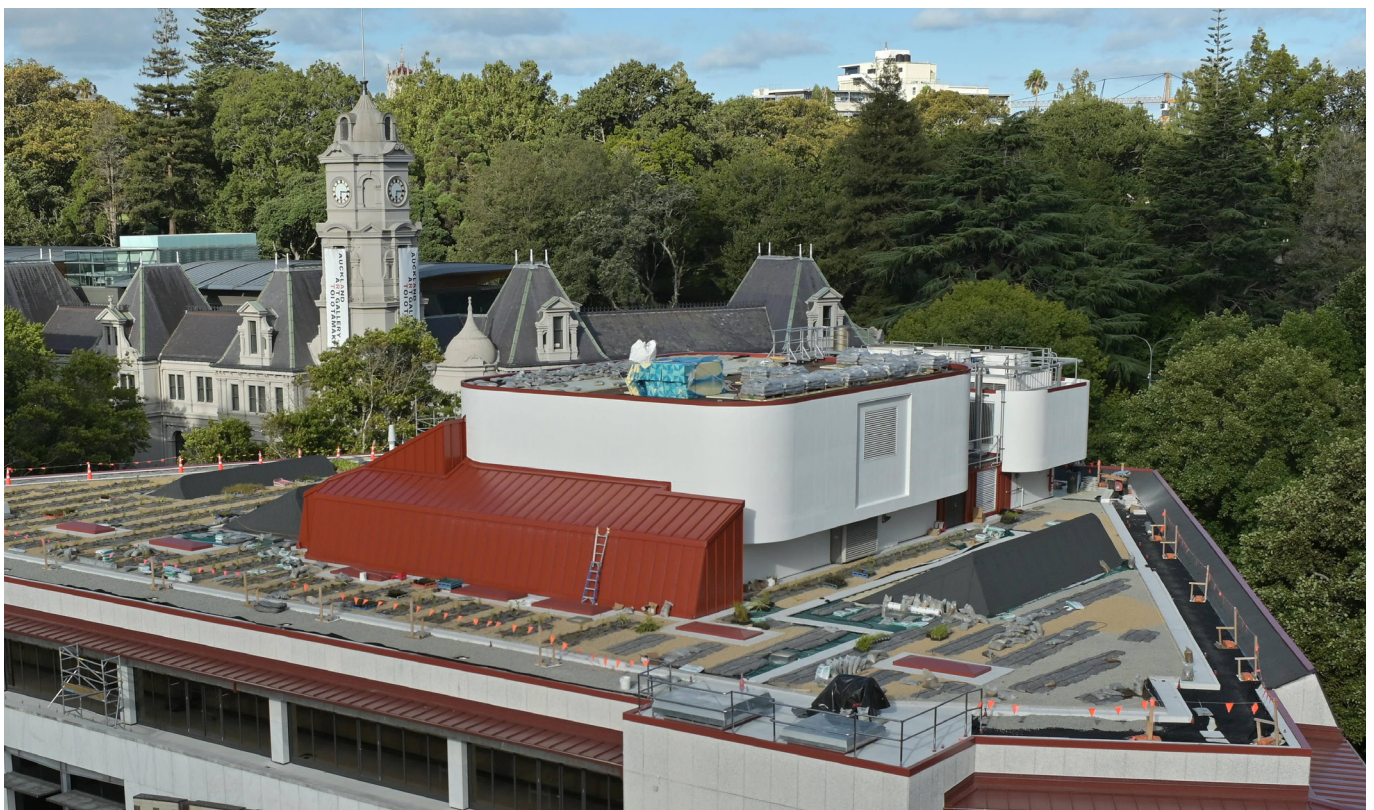
Figure 5: Auckland Central Library living roof under construction Source: Timescapes Limited
