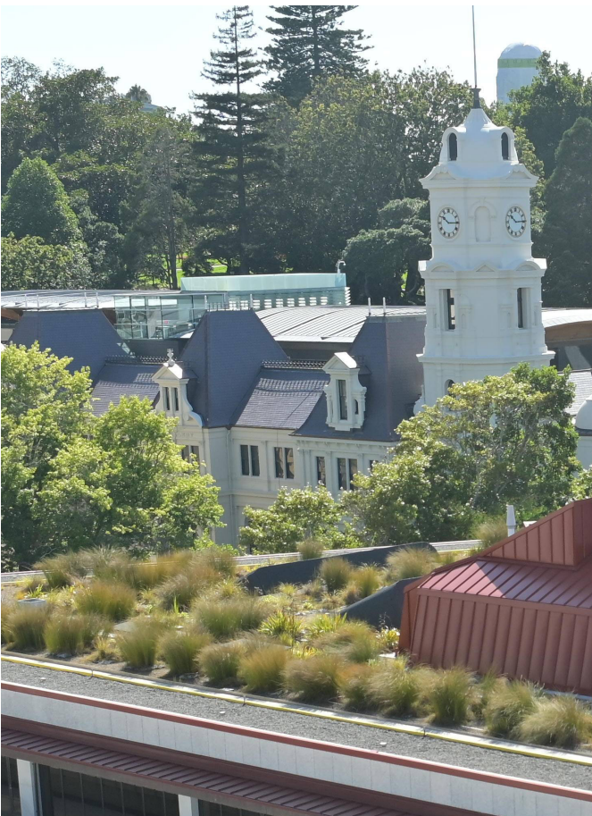
Figure 25: Auckland Central Library living roof Source: Timescapes Limited
