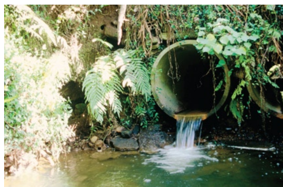
FIGURE 8 Example of a perched culvert, a common barrier to fish passage. Native fish are unable to leap the vertical distance required to enter the culvert and continue migrating upstream. (Source: ARC).
